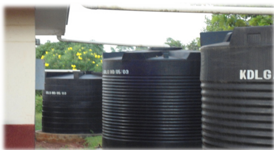
Figure 5: Rain water harvesting at Bupadhengo HCII
