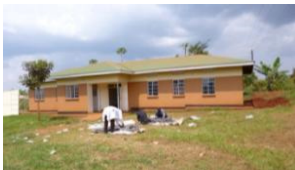
Figure 4: A newly constructed maternity ward at Budondo HCIII
