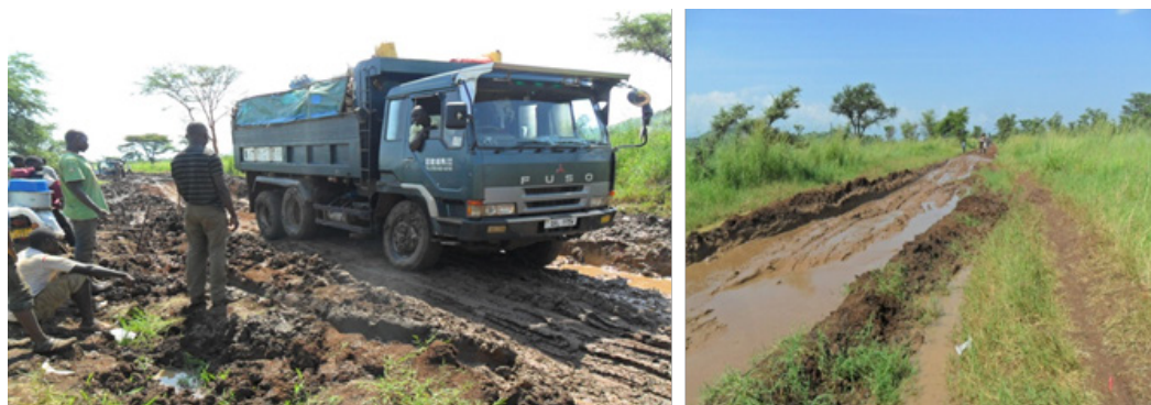
Figure 3: Effect of Marble-carrying trucks on Nakapiripirit-Mbale Road
