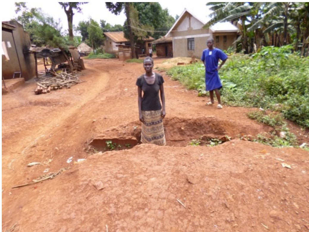
Figure 7: Sakabusolo road, in Mafubira Sub-county
