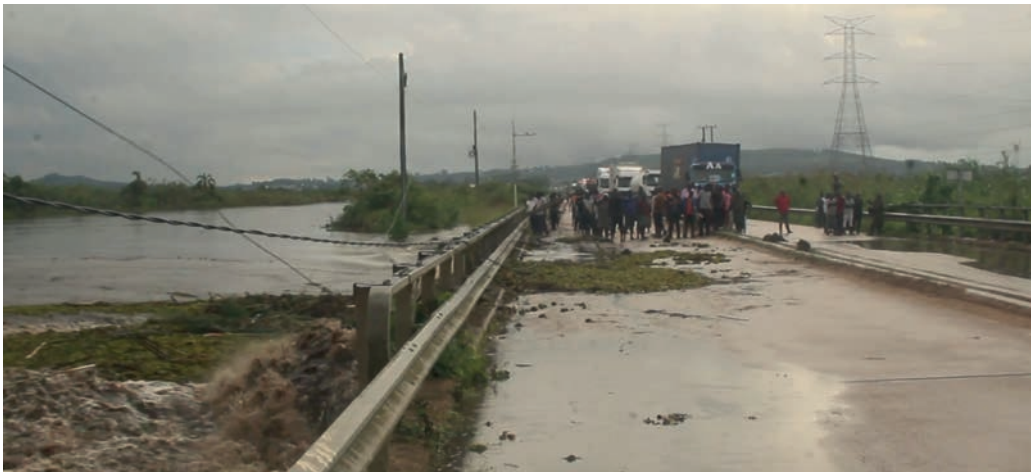
Residents watching Kotonga bridge along Mbarara - Masaka highway that was washed away by flash floods in May, 2023
