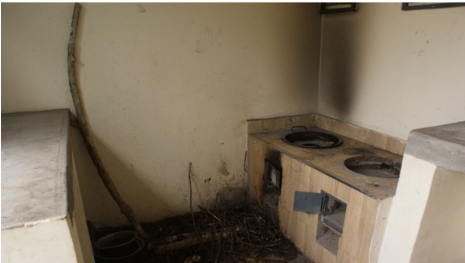
Figure 14: An Energy saving stove at one of the PAPs House Hold in Kyotera
